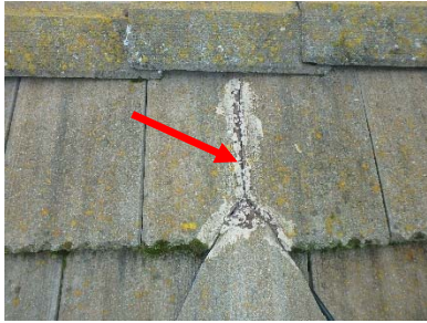
Cracked Adhesive
