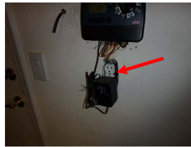
Right Side Garage Wall
