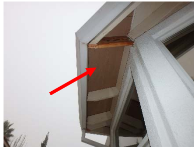
Roof Sheathing @ Rear
