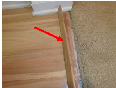
Loose Threshold Piece
